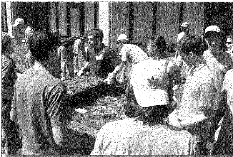
Students Installing Modular Trays for a Green Roof At University of Connecticut
